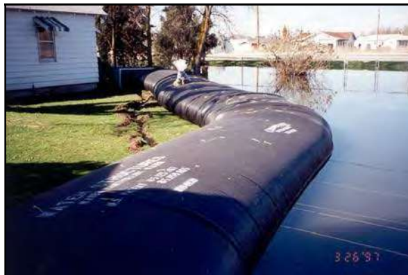
More 3' and 4' high AquaDams® used for flood protection in Sun Valley, ID.
