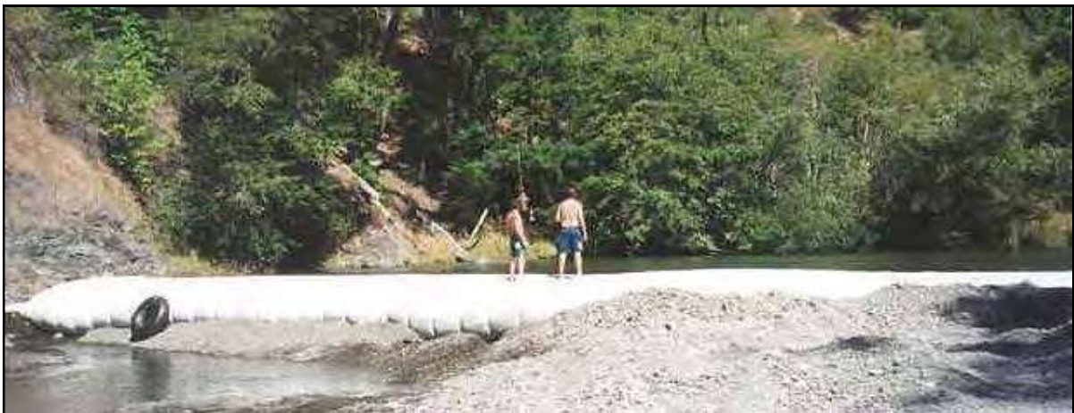
A 5' high AquaDam® installed in Larabee Creek, CA to contain water for a swimming hole.
