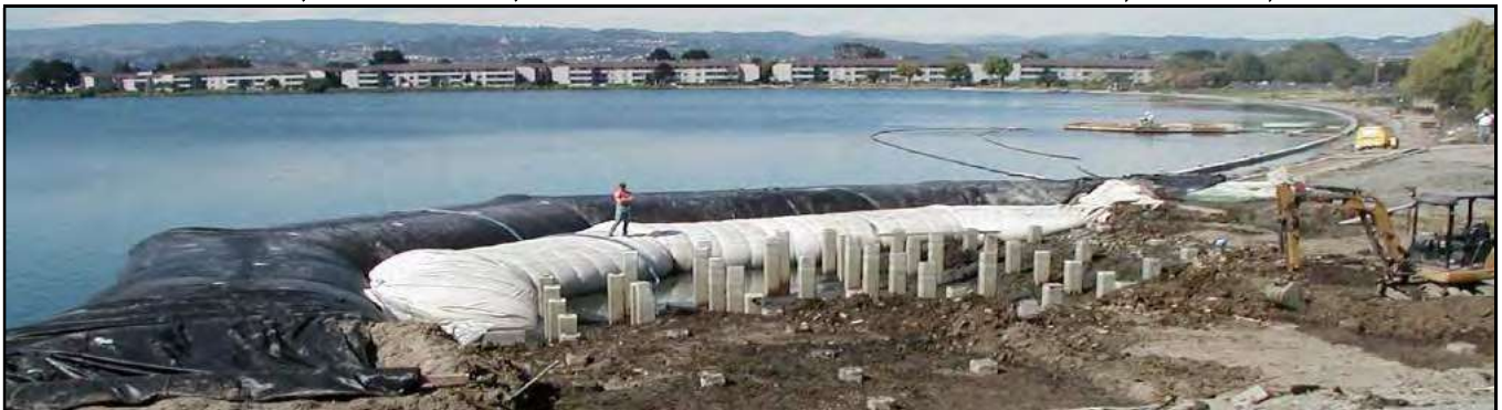
Dewatering for amphitheater construction, Foster City, CA.
