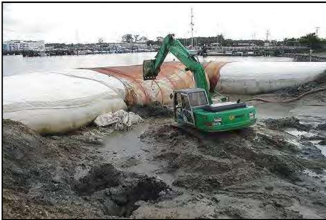
16' high AquaDam® at Little Creek Naval Amphibious Base. Norfolk, VA
