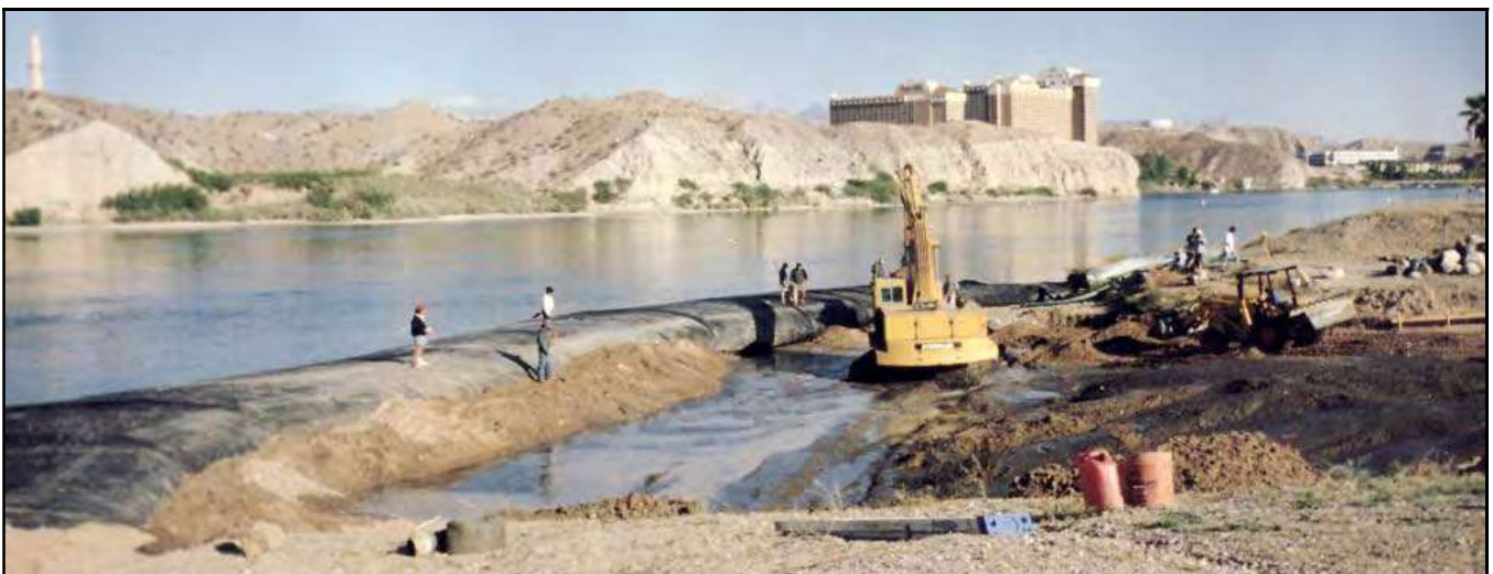
9' high AquaDam® used for boat ramp construction in Bullhead City, CA.
