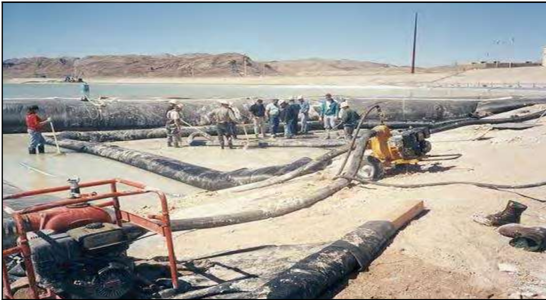
1,300 linear feet of AquaDams® in an arsenic pond, Northern WA.
