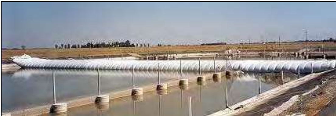
7' high AquaDam® used to split a sanitation pond in Yolo County, CA.
