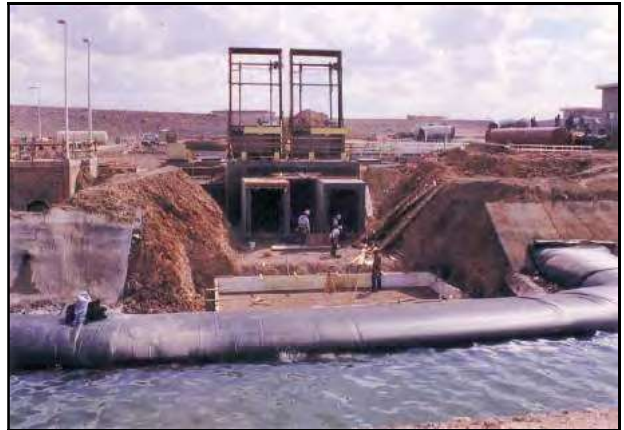
AquaDams® used to dewater a canal bank on the Salt River Project. Phoenix, AZ.
