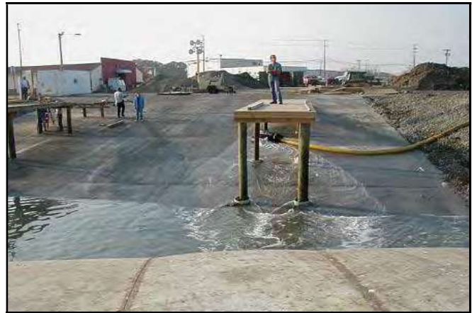
16' high AquaDam® at Little Creek Naval Amphibious Base. Norfolk, VA
