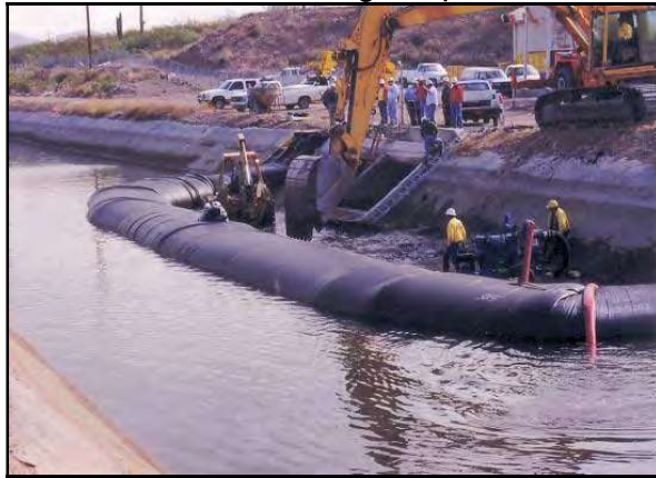
AquaDams® used to dewater a canal bank on the Salt River Project. Phoenix, AZ.
