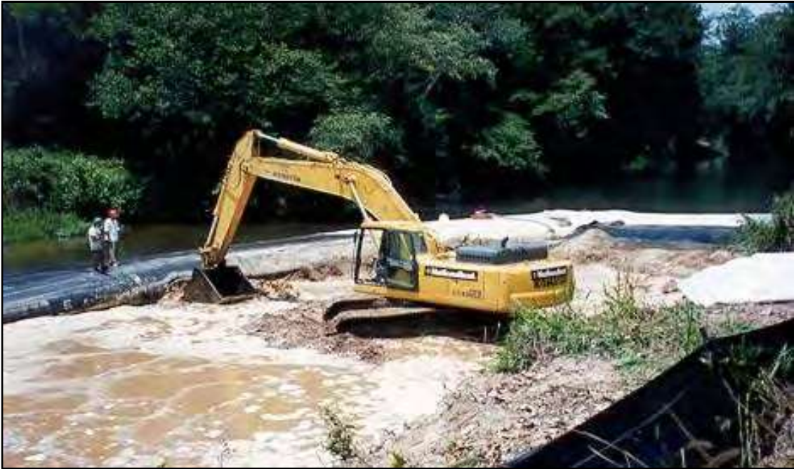
8', 6' and 4' high AquaDams® used to contain sediments during a Williams Transco natural gas pipeline repair project on the Bogue Chitto River. McComb, Mississippi.
