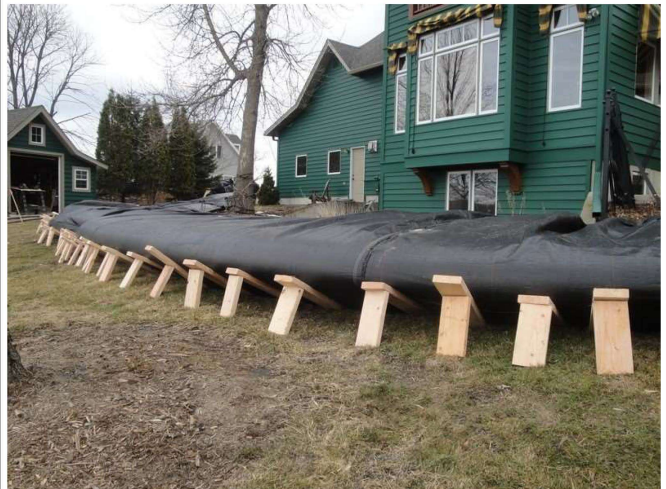
Many 2-board braces are in place along the side of the partially filled AquaDam, in the area it is running parallel to the bank.
