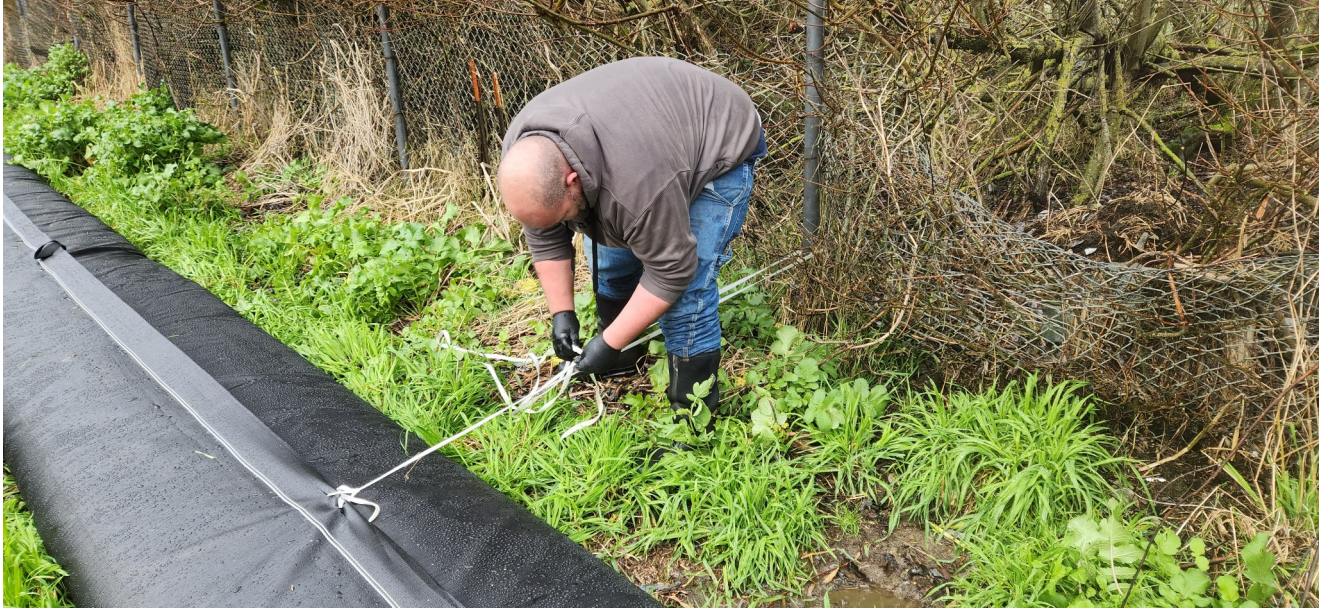
Image 13: The AquaDam can be tied to anchor points to help keep the unit from rolling/sliding on cross slopes.
