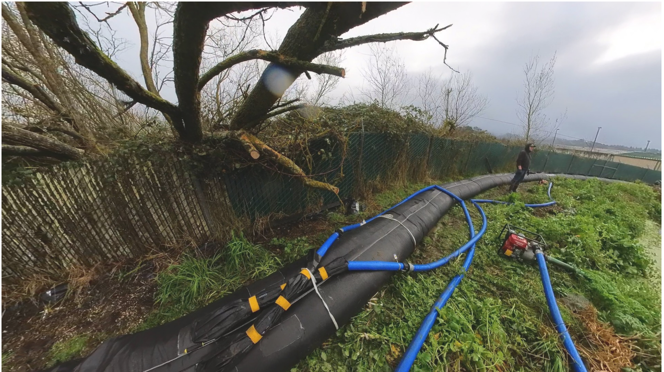
Image 10: SCE AquaDam filling using two (2) 3" Honda WB30XT water pumps.
