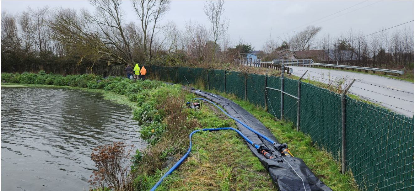
Image 4: 1.5' tall double closed end (DCE) Starter AquaDam being filled using the wastewater on site.
