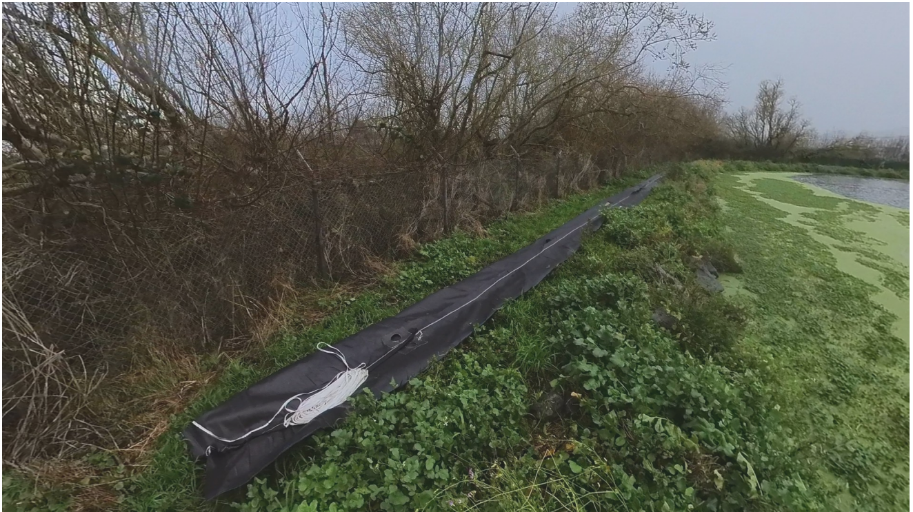
Image 9: SCE AquaDam at the end with a connection collar.
