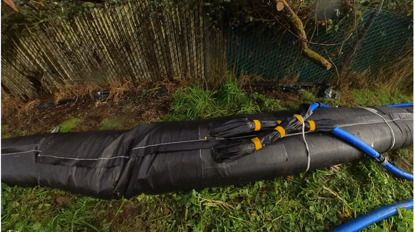
Image 11: Top view of the two AquaDams connected with a connection collar and the second AquaDam filling.
