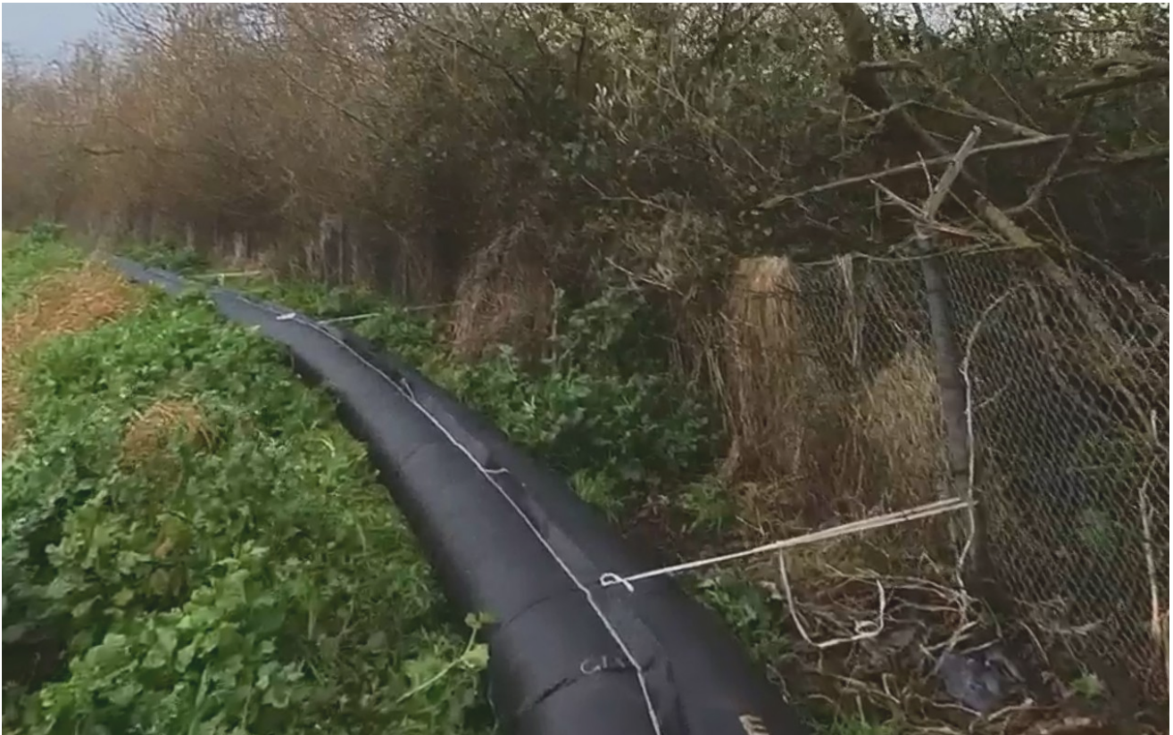
Image 14: AquaDams can be tied back at multiple points to keep from rolling on a cross slope.
