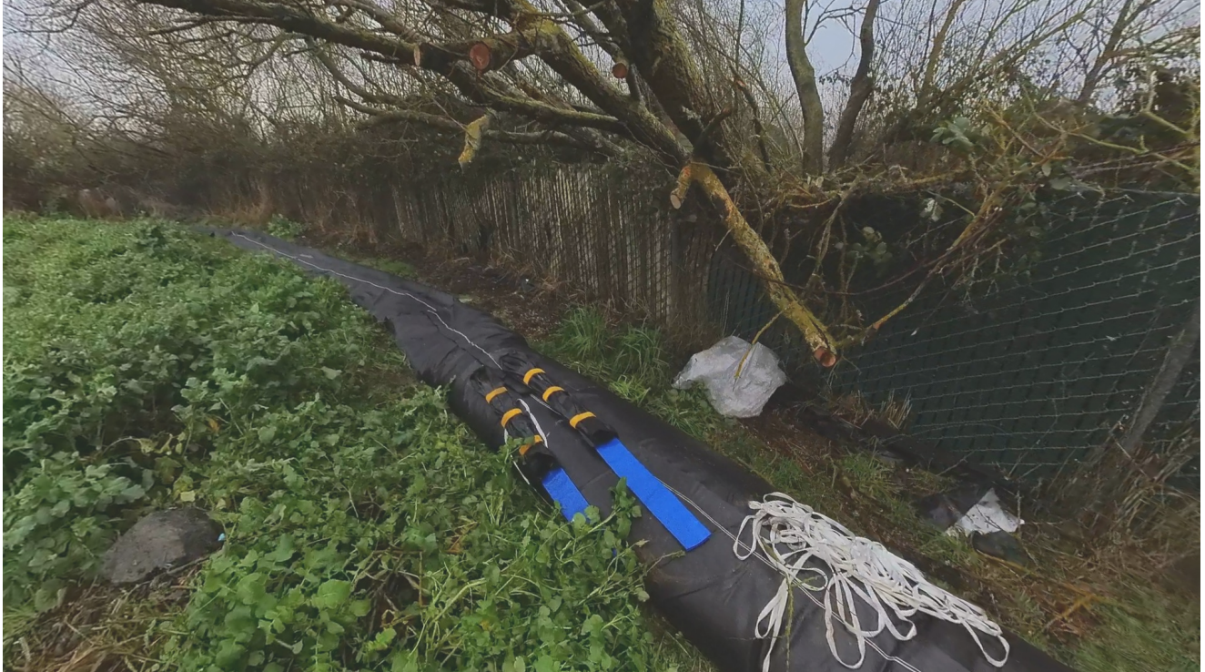
Image 8: A single closed end (SCE) AquaDam has been connected to the DCE AquaDam with the connection collar prior to the DCE AquaDam being full.
