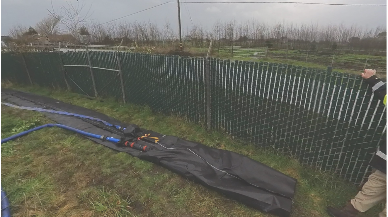
Image 5: Pumping both fill tubes of the DCE AquaDam with two connection collars.
