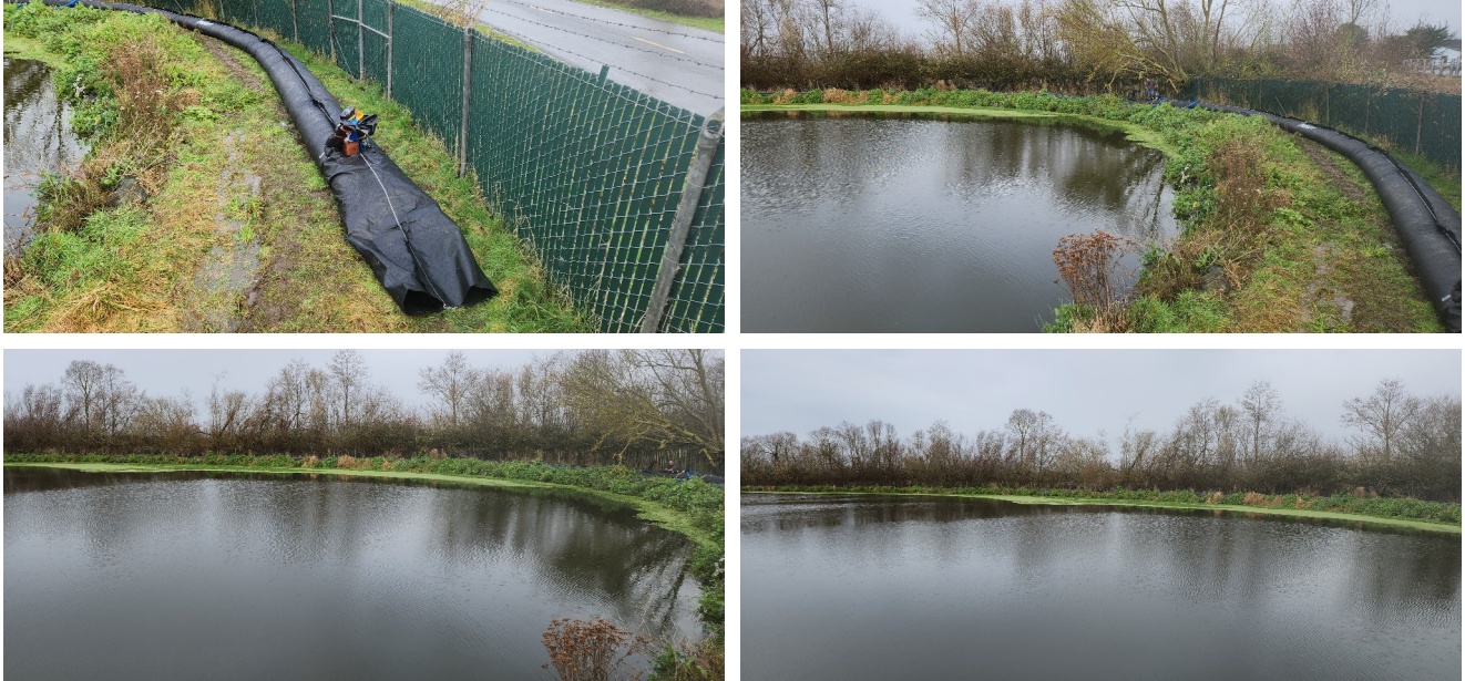
Image 15: Four photos of AquaDams installed around the pond.
