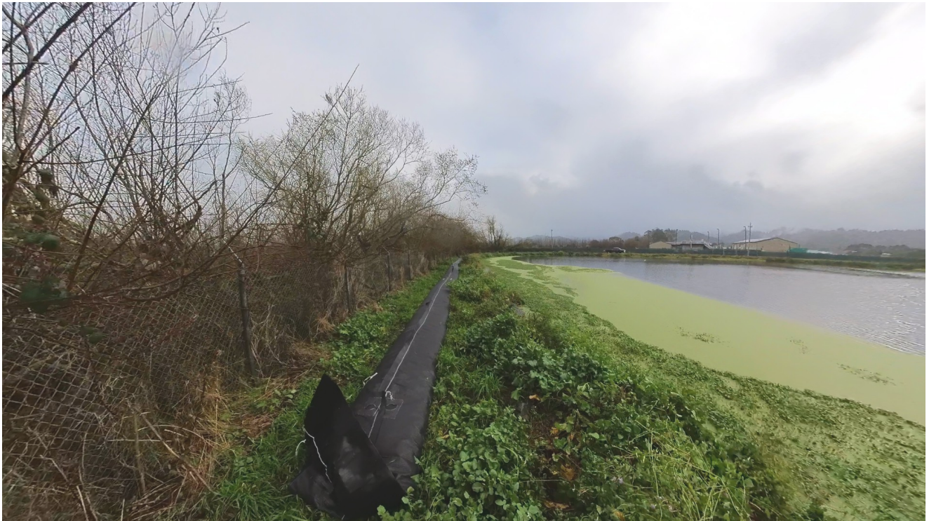
Image 12: End of SCE AquaDam with connection collar ready for the next AquaDam, if extra length is needed.
