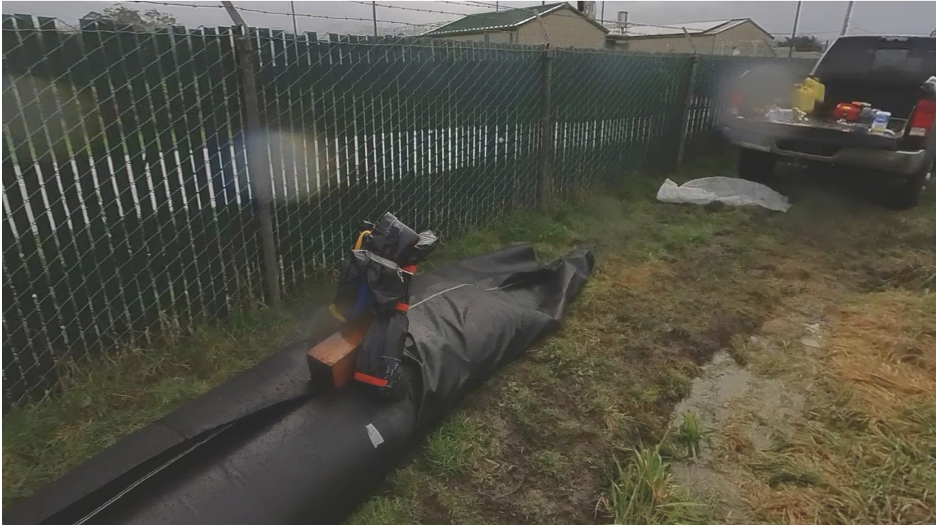
Image 7: The fill tube on the AquaDam have been reinforced and elevated to keep the water inside secured.
