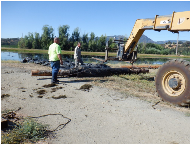
AquaDam re-roll with one piece of timber (notice the angle in ropes).
