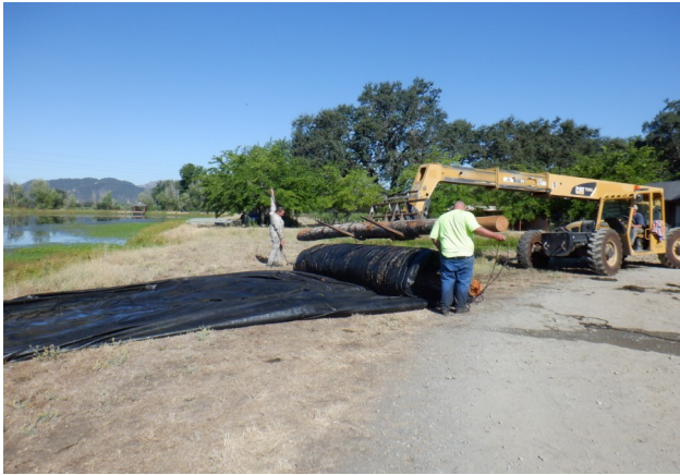
Dual timber re-roll example.
