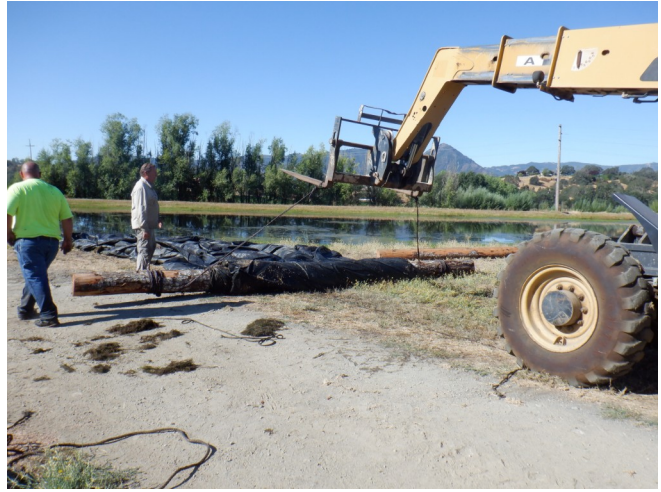
AquaDam re-roll with one piece of timber (notice the angle in ropes).
