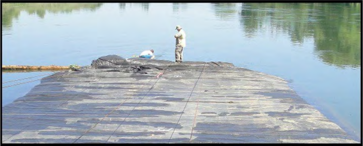
Figure 5: Using Ropes to Install an AquaDam® in Flowing Water
